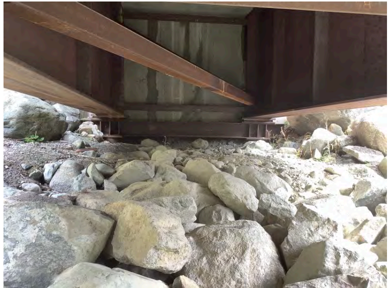
Left Bank Abutment when facing downstream
