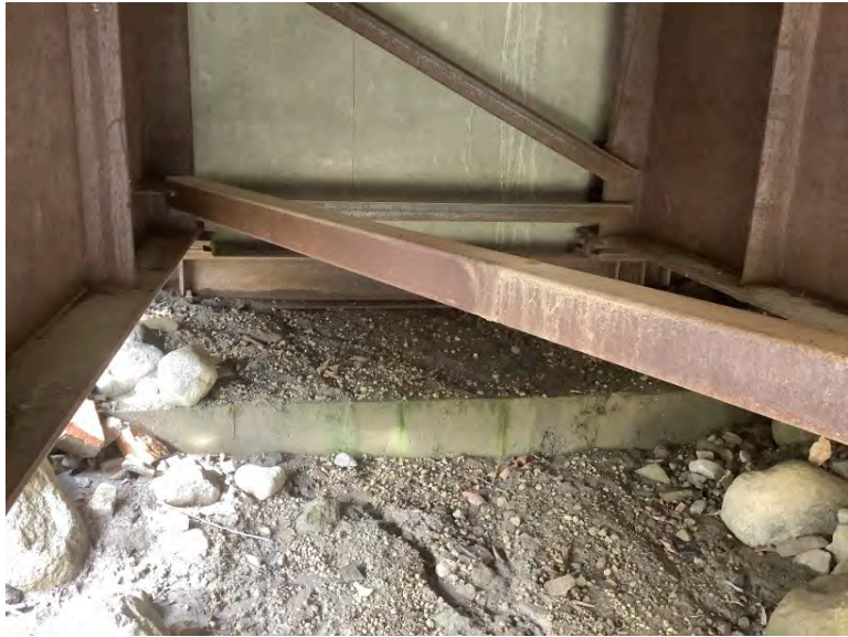
Right Bank Abutment when facing downstream
