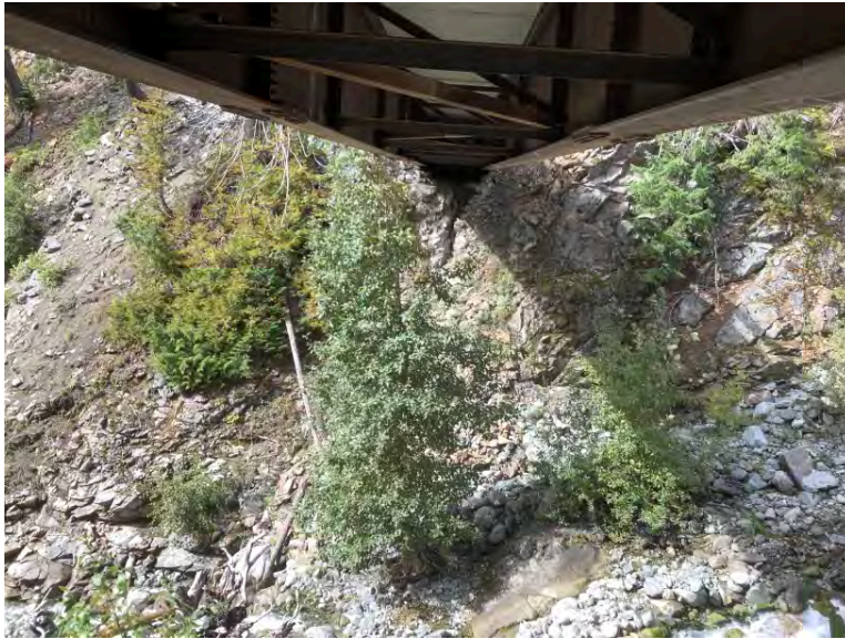
Right Bank Abutment when facing downstream
